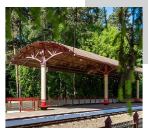
Railways Platform Sheds
