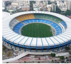
Stadium Roofing System
